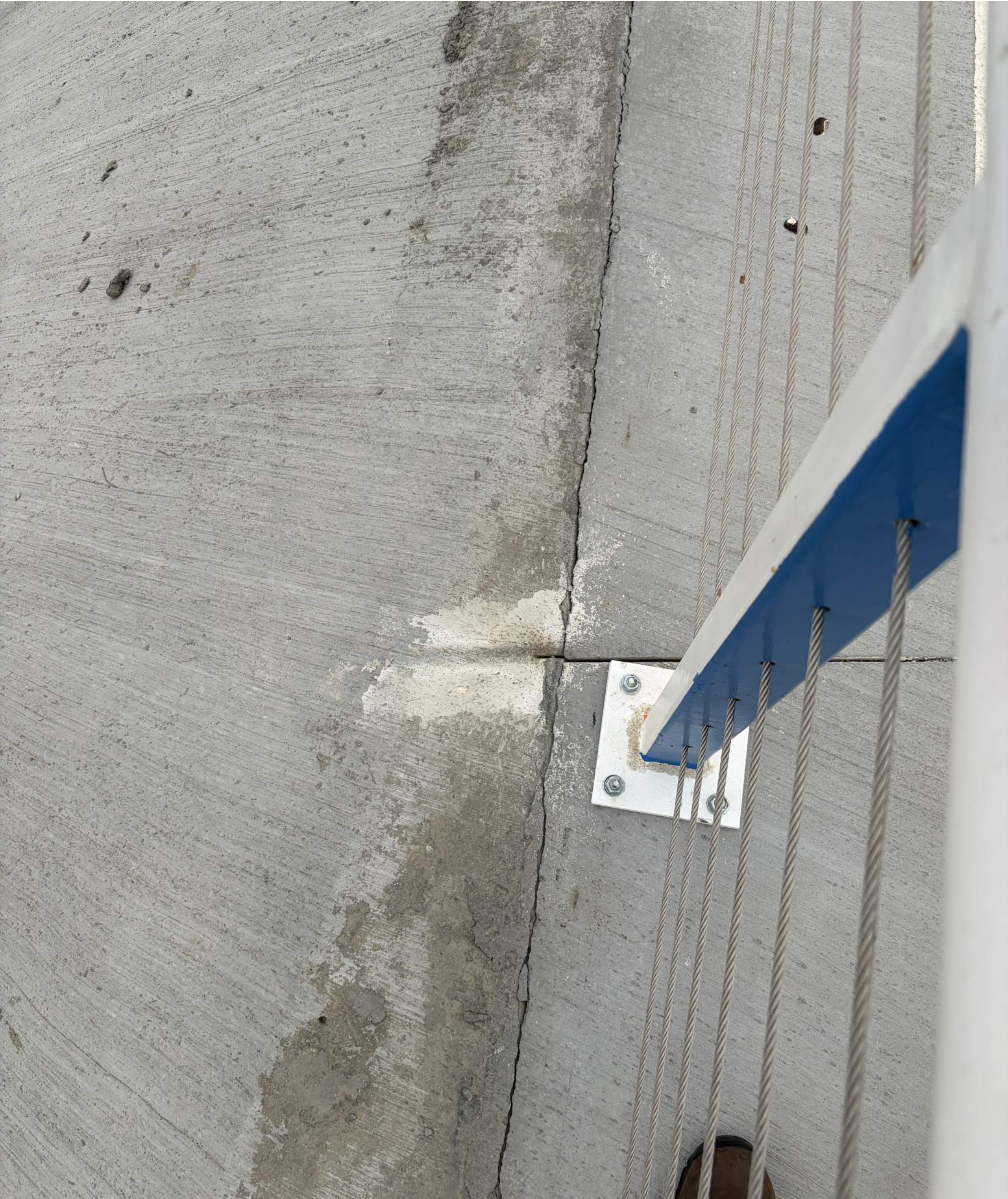
PHOTOGRAPH 4 - BASE PLATE AT JEFFERSON STREET
