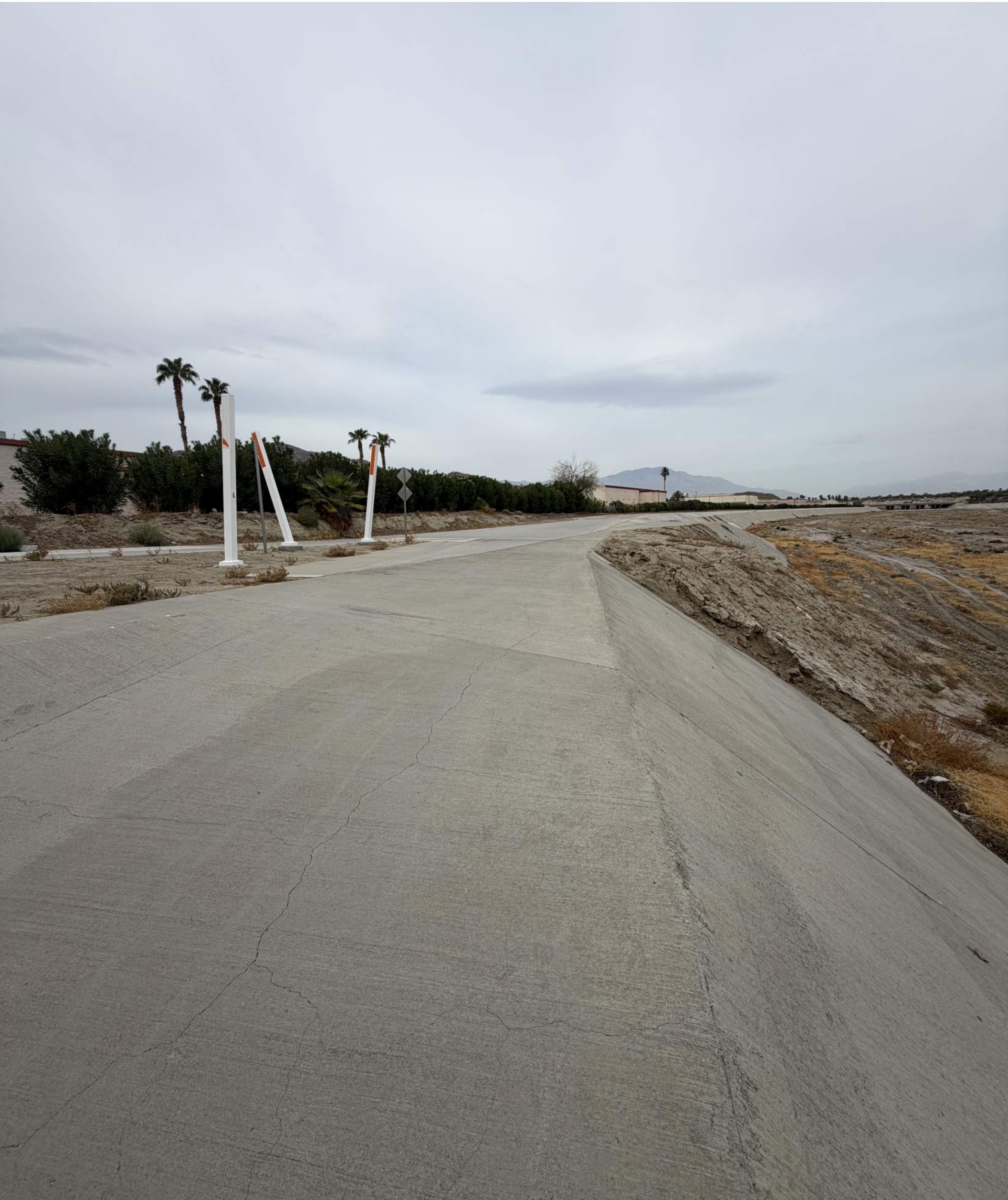
PHOTOGRAPH 2 - WEST OF ADAMS STREET UNDERCROSSING, LOOKING WEST
