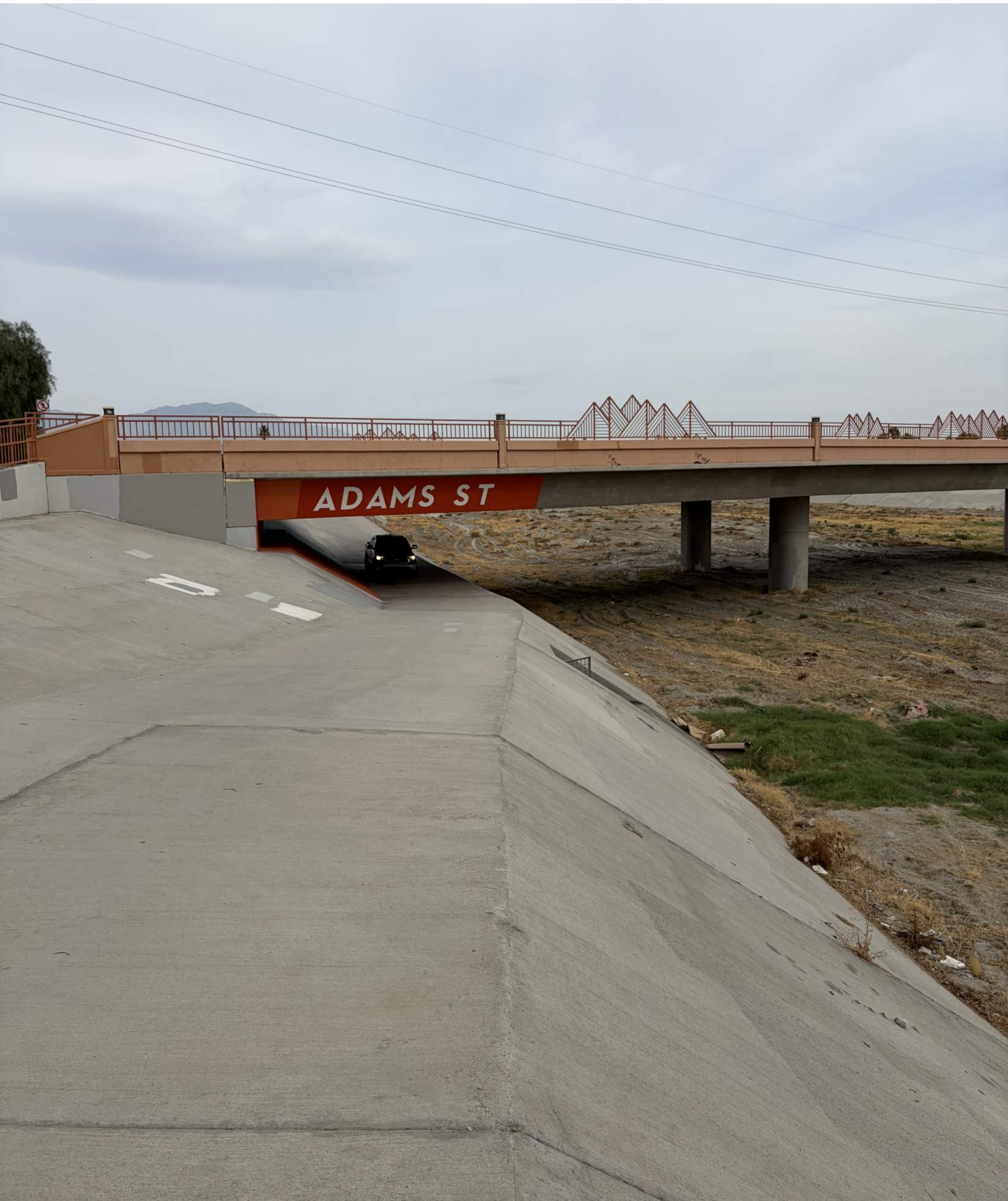
PHOTOGRAPH 1 - ADAMS STREET UNDERCROSSING LOOKING WEST
