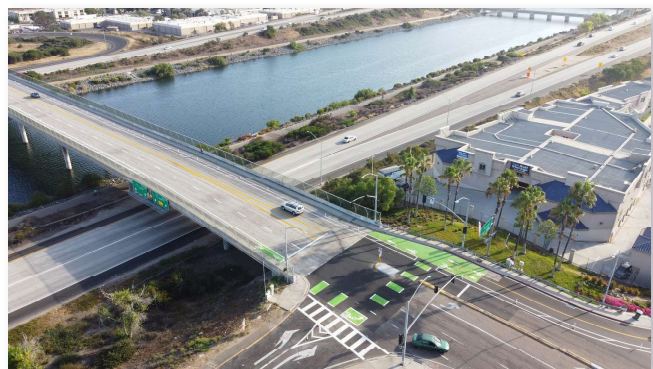
Bikeway crossing freeway (CRA designed project in National City)
