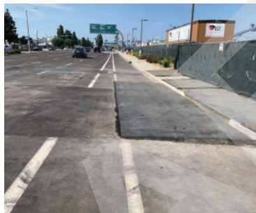
Construction Plating Installed Within a Bike Lane
