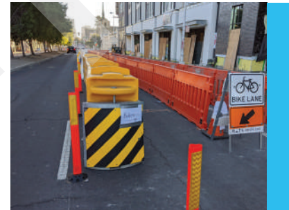
Temporary Separated Bicycle Path Behind Barrier
