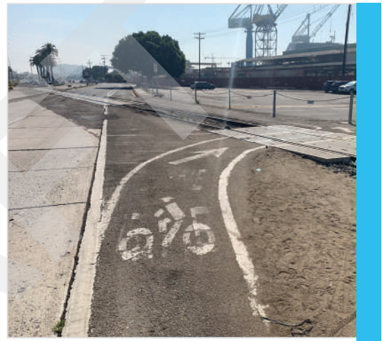
Bike Lane Designed to Cross Perpendicular to Railroad Crossing
