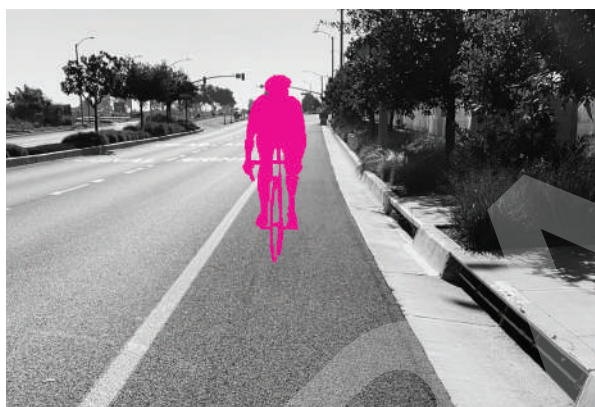
Catch Basin Without Extended Local Depression
