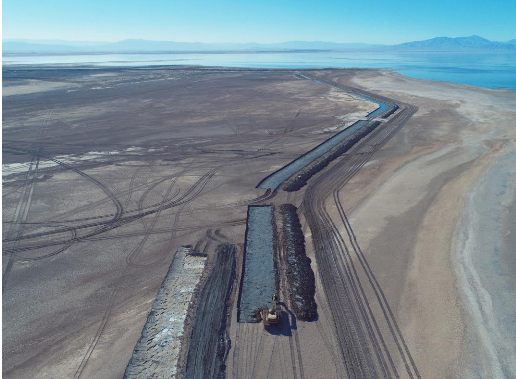
Excavation of deep channel along northern berm of habitat pond
