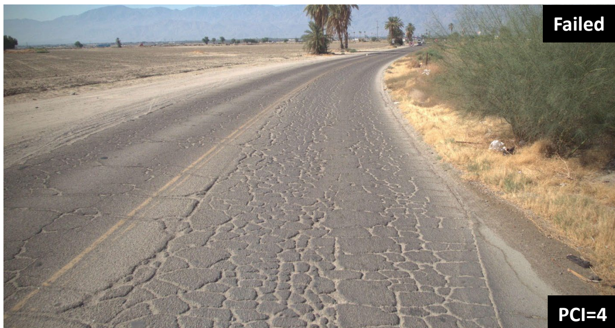
Figure 13: Section of Dillon Road in Failed Condition
