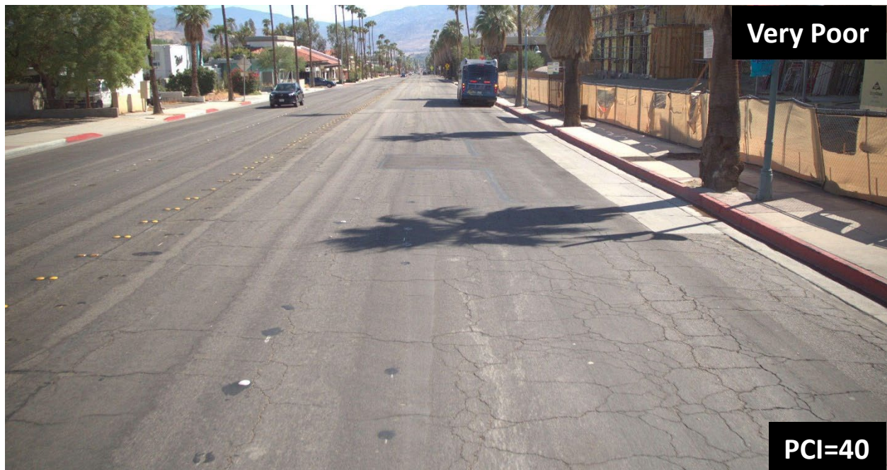
Figure 11: Section of North Palm Canyon Drive in Very Poor Condition
