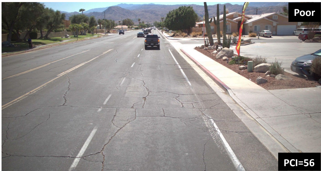
Figure 10: Section of Cathedral Canyon Drive in Poor Condition
