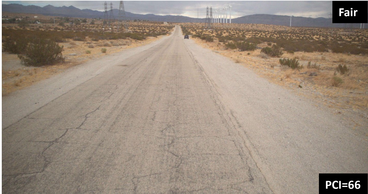
Figure 9: Section of Worsley Road in Fair Condition
