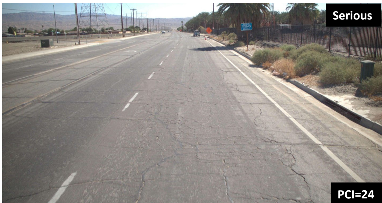
Figure 12: Section of Avenue 52 in Serious Condition
