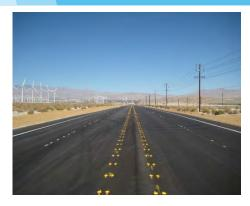
Dokken completed preliminary environmental engineering, document, PS&E and construction management services for the widening of Indian Canyon Drive from two lanes to four lanes through the Whitewater River wash. The engineering design studies assisted in providing a scour protection measure, avoiding conflicts. utility determining right of
